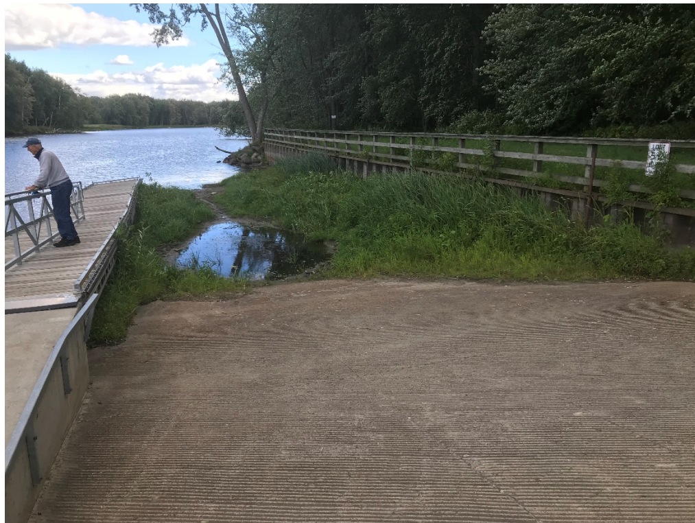
Figure 4. Severe siltation issues on the Colchester Point Fishing Access Area ramp on the Winooski River in Colchester Point.
